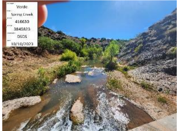
Figure 153. Downstream to downstream view of SPC14-F, Spring Creek, Arizona.
