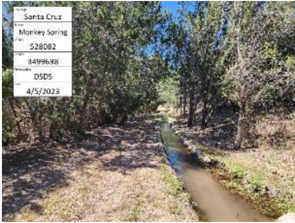
Figure 93. Downstream to downstream view of MKS01-F, Monkey Spring, Arizona.
