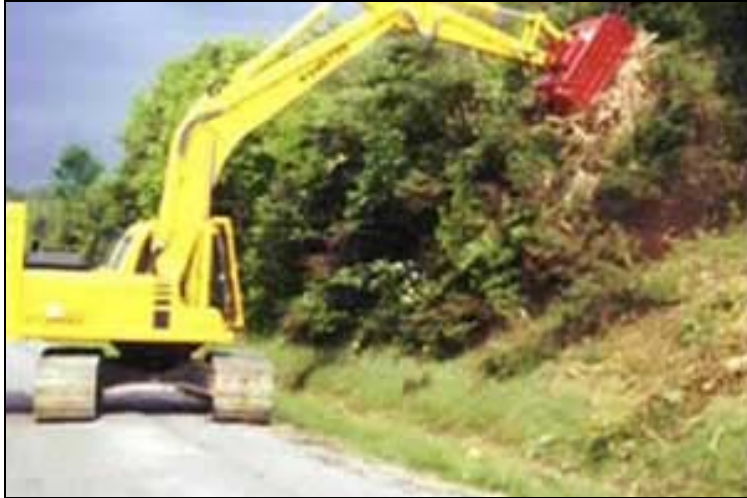
Figure 4. Excavator with Fecon head clearing roadside slope.
