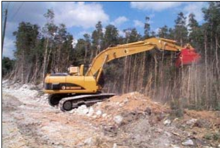
Figure 3. Excavator with Fecon head clearing dog-hair thicket.
