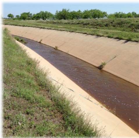
Bretch Canal, Mountain Park Project.
