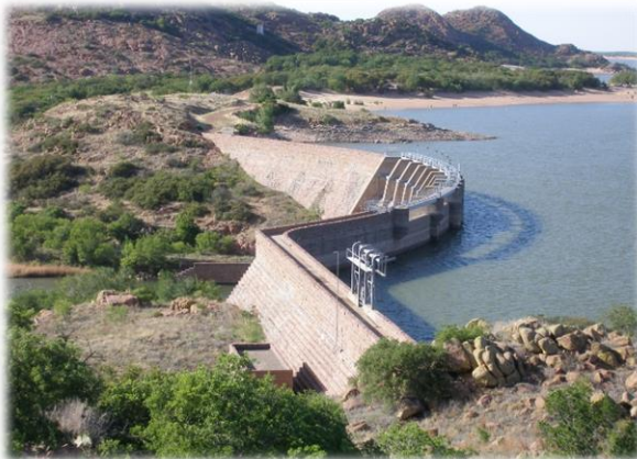
Altus Dam, Lugert-Altus Reservoir.
