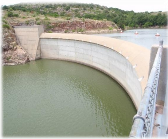
Mountain Park Dam, Mountain Park Project.
