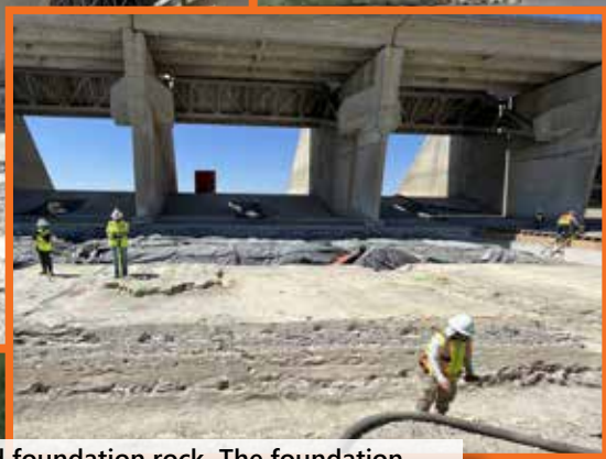
Reclamation geologists map exposed foundation rock. The foundation must be mapped and approved by geologists in order to identify any geologic features that could affect the performance of the new structure and may require mitigation. Examples would be faults or fractures, loose blocks of material, sharp overhangs and bentonite seams.
