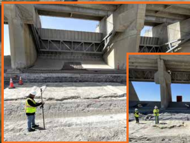
Reclamation geologists map exposed foundation rock. The foundation must be mapped and approved by geologists in order to identify any geologic features that could affect the performance of the new structure and may require mitigation. Examples would be faults or fractures, loose blocks of material, sharp overhangs and bentonite seams.
