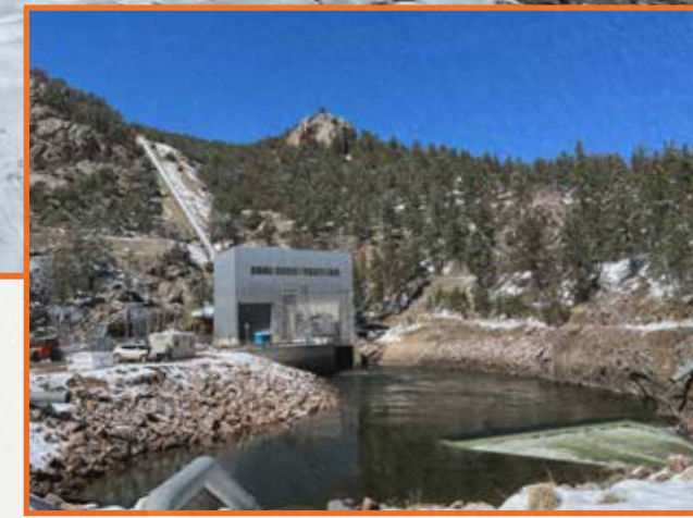
Grout plant setup on the afterbay dam. The plant operator stays in radio and visual contact with the nozzleman working in the outlet structure to contact grout below the existing slab. Photo by Tom Hastings.
