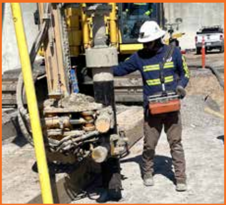
Contractor aligns casing and prepares to drill borehole for anchor bar for new spillway slab. Rock anchors are steel bars that are set into boreholes and grouted, providing a solid connection to the foundation for the new spillway slab.
