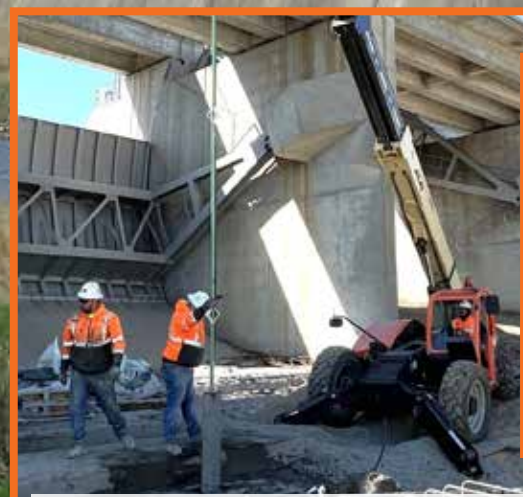
Contractor aligns casing and prepares to drill borehole for anchor bar for new spillway slab. Rock anchors are steel bars that are set into boreholes and grouted, providing a solid connection to the foundation for the new spillway slab.
