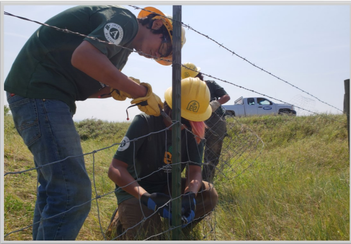
(Above) Montana Conservation Corp boundary fence project.
