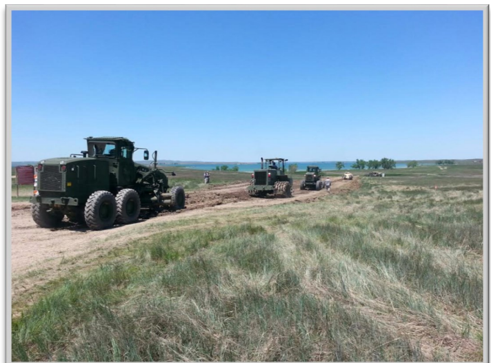
(Above) South Dakota Army National Guard constructing Bird Island View Road.
