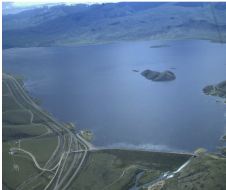
Figure 13.—MTG - Aerial view of Clark Canyon Reservoir.
