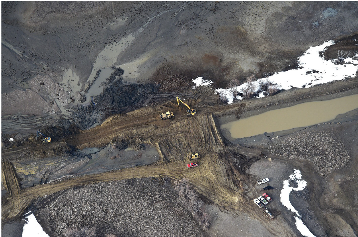
Figure 31.—MTG - Malta Irrigation District repairing Dodson South Canal, April 2023.
