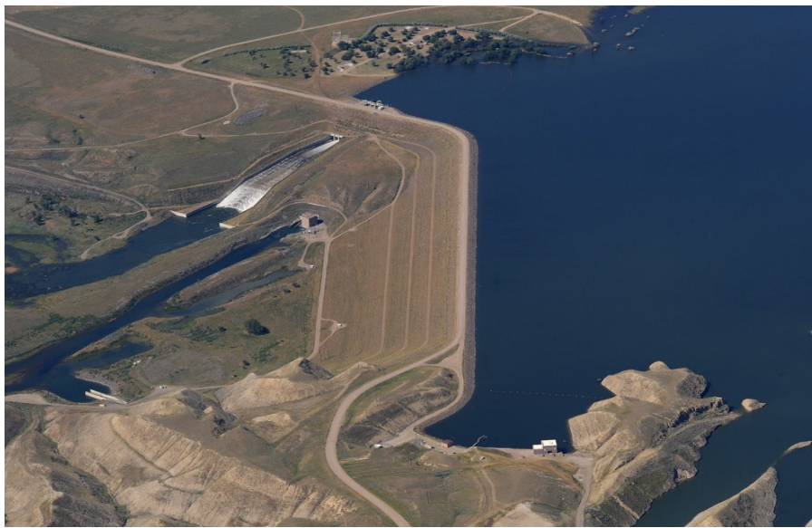
Figure 27.—MTG - View of Tiber Dam and Lake Elwell.
