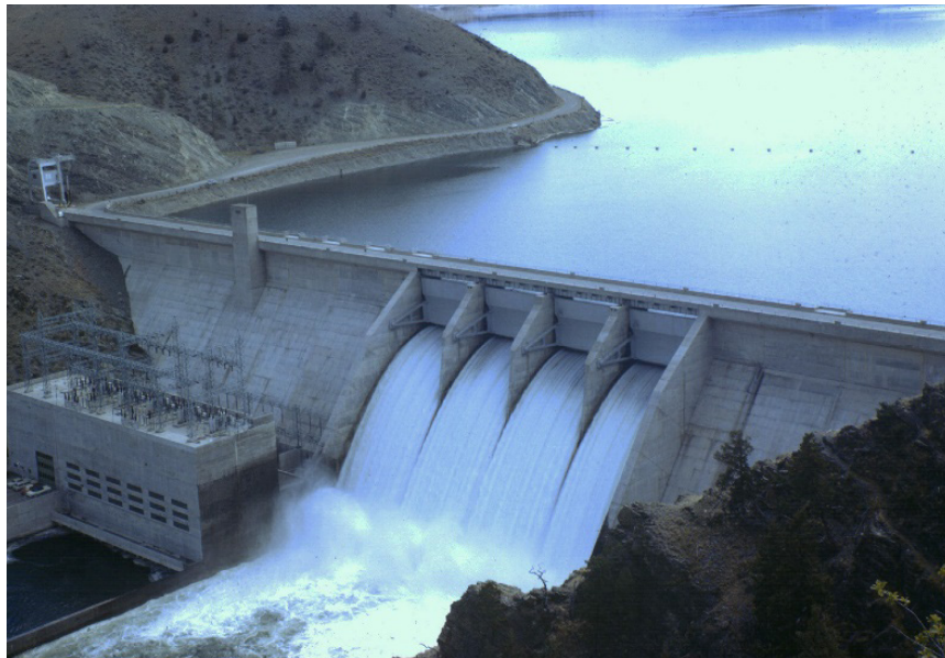
Figure 16.—MTG. - Canyon Ferry Dam and Powerplant.
