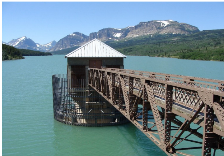
Figure 29.—MTG - Lake Sherburne's outlet works.
