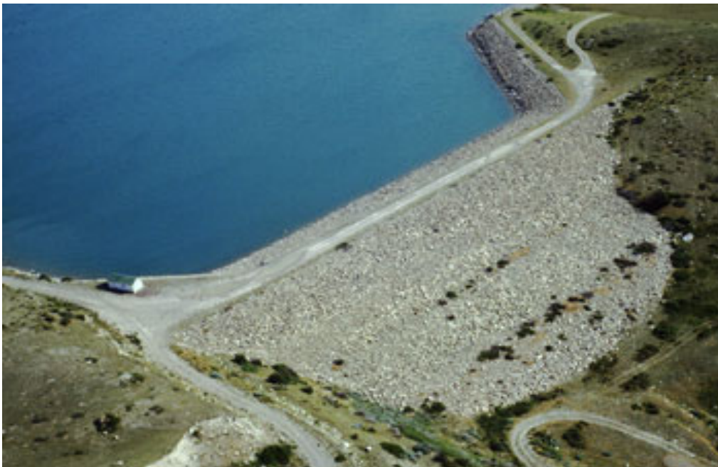
Figure 23.—MTG - View of Willow Creek Dam and Reservoir.
