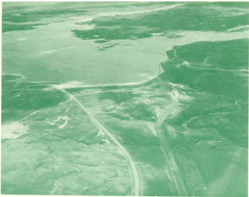
Merritt Dam & Reservoir
