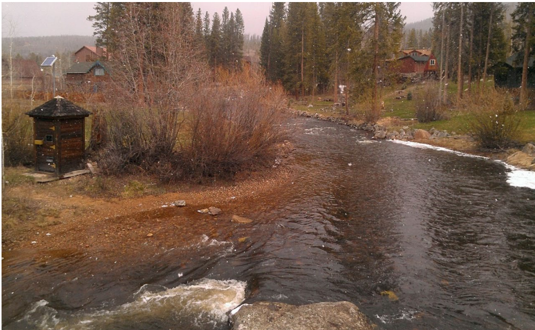
Figure 4.—North Inlet near Grand Lake. Stream gaging house is shown on left side of photo.
