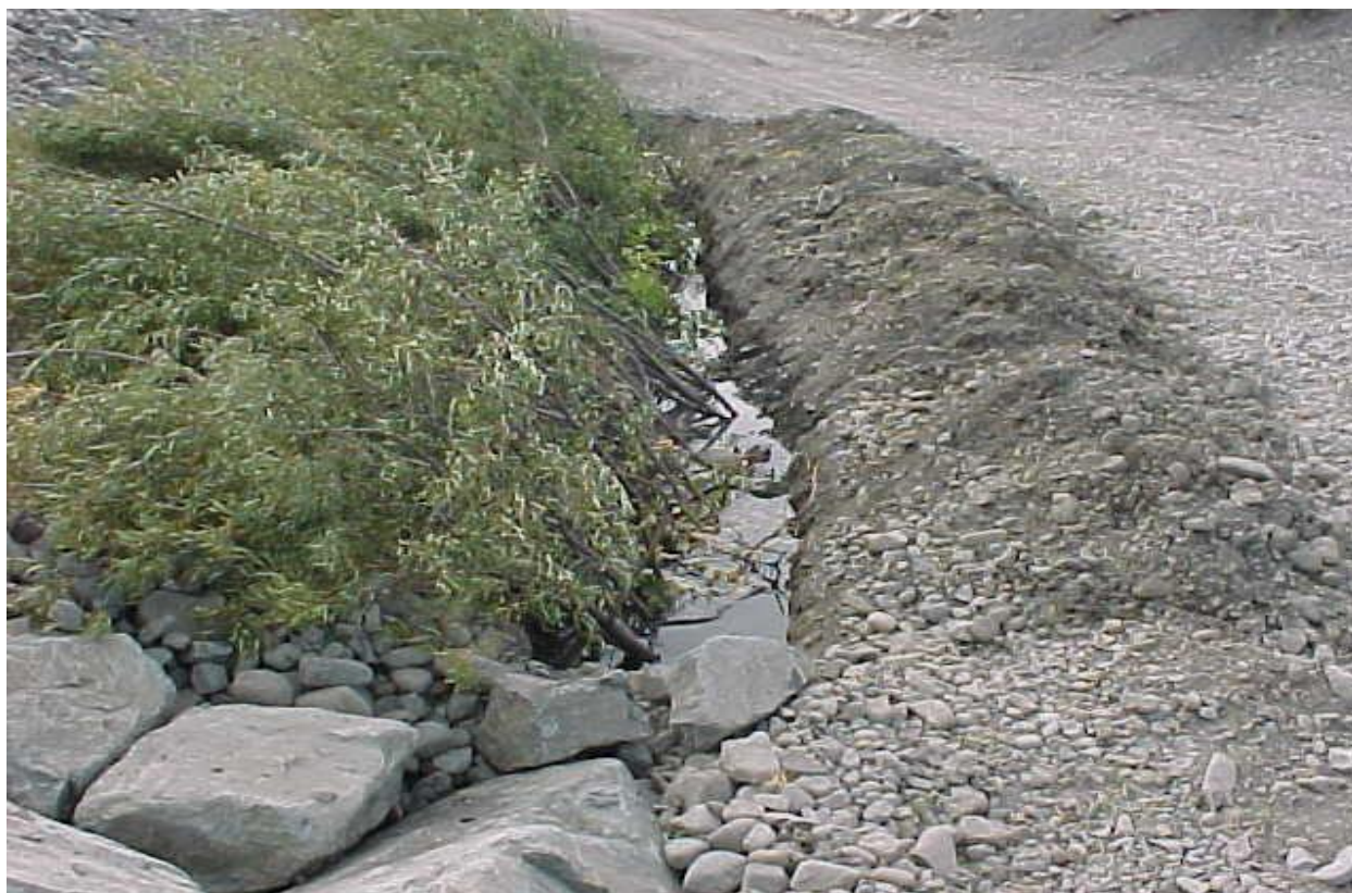
Picture 5. Willow Wall planted in wetted trench adjacent to point where water flow goes subterranean.
