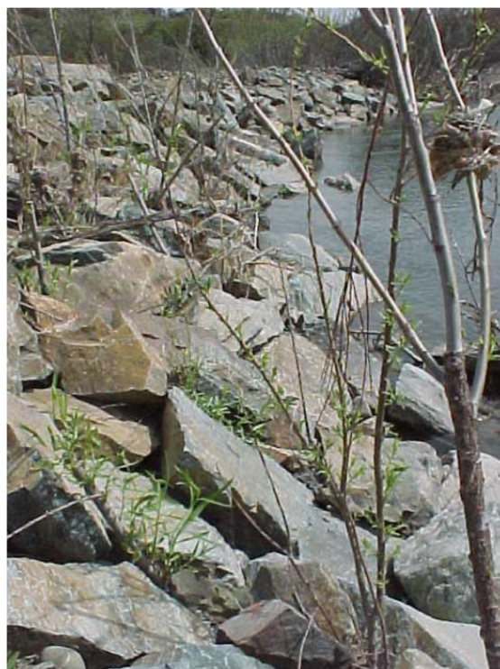
Picture 4. Interstitial Sprigging.
