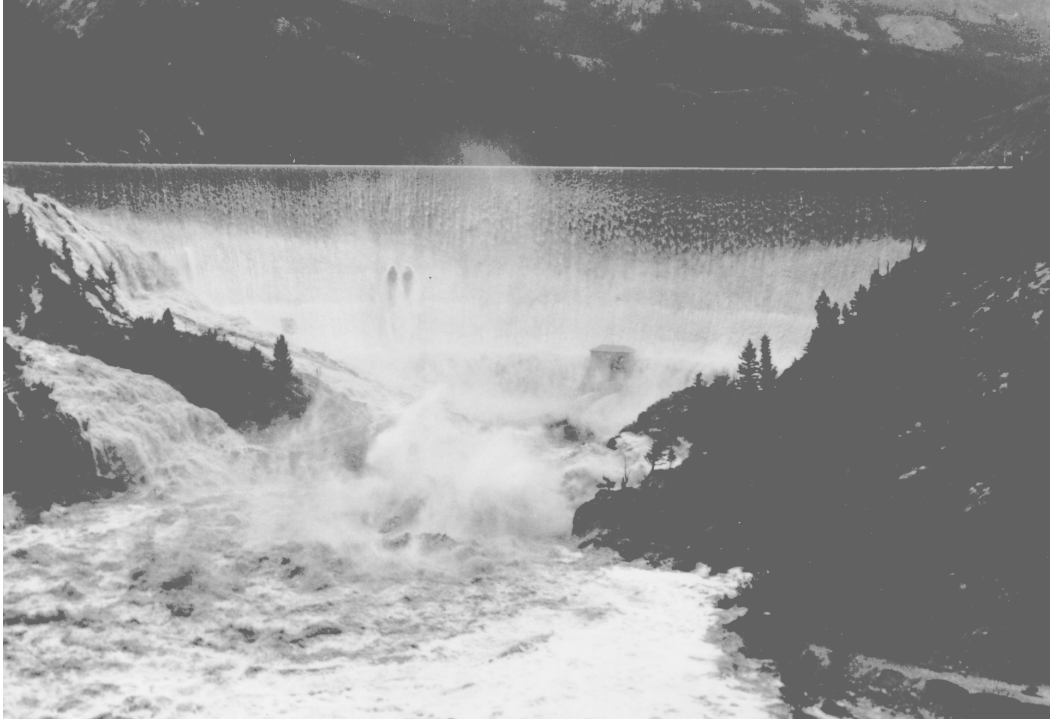
Figure GM-2. Overtopping of Gibson Dam in 1964
