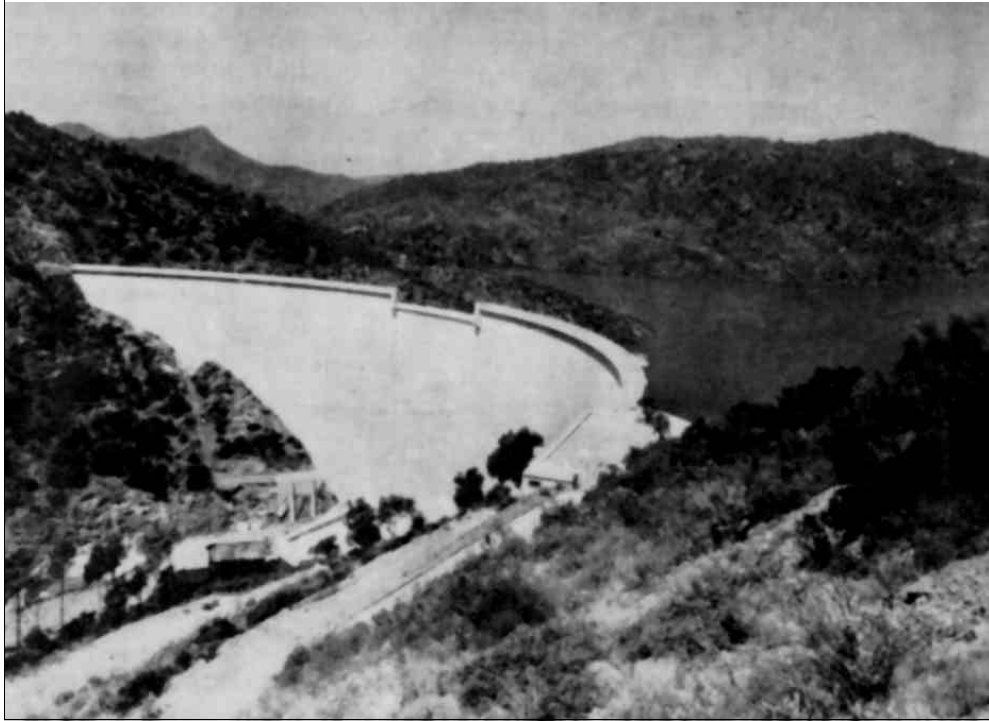
Figure MF-3. Malpasset Dam before failure (after Bellier, 1967)
