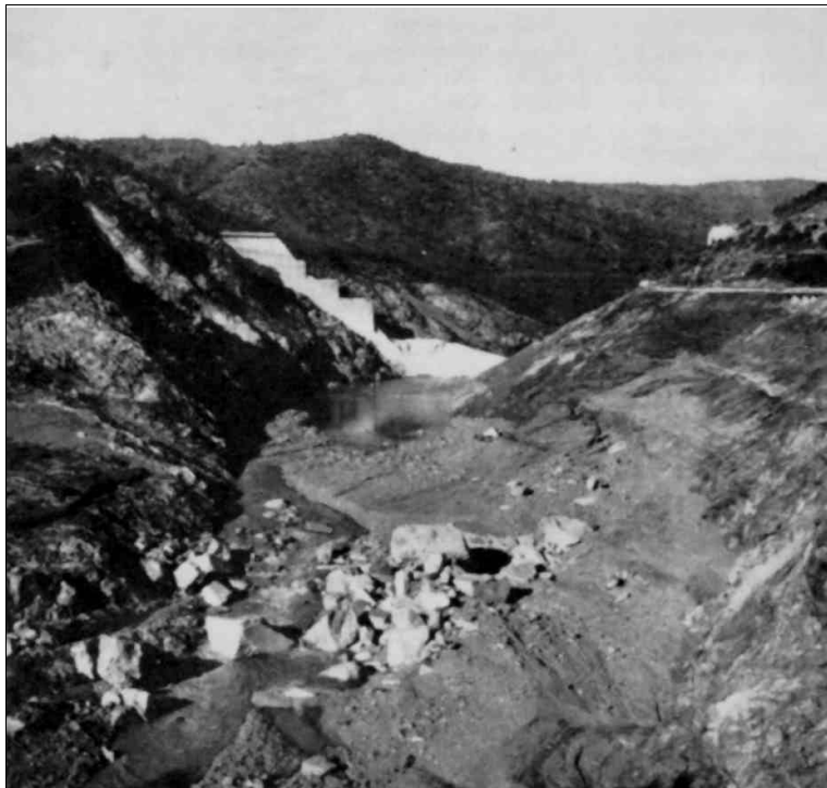
Figure MP-6. Looking from downstream after failure (after Bellier, 1967)
