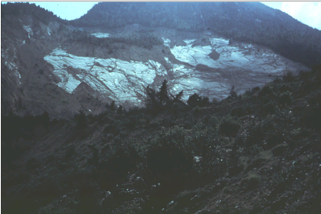
Figure VI-2. View of left reservoir bank following failure
