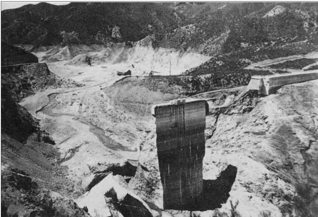
Figure SC-3. St. Francis Dam after the failure (Huber Collection, U of Cal Water Res Center Archives)
