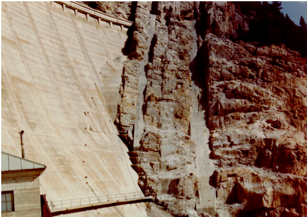
Figure GM-3. Overtopping protection on left abutment
