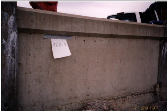
Type IV cement, mix 42B, panel 4
