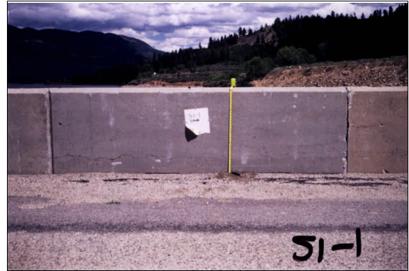
Type V cement, mix 51, panel 1
