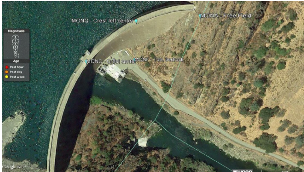
Figure 14. Aerial View of Monticello Dam and Seismic Instrumentation
