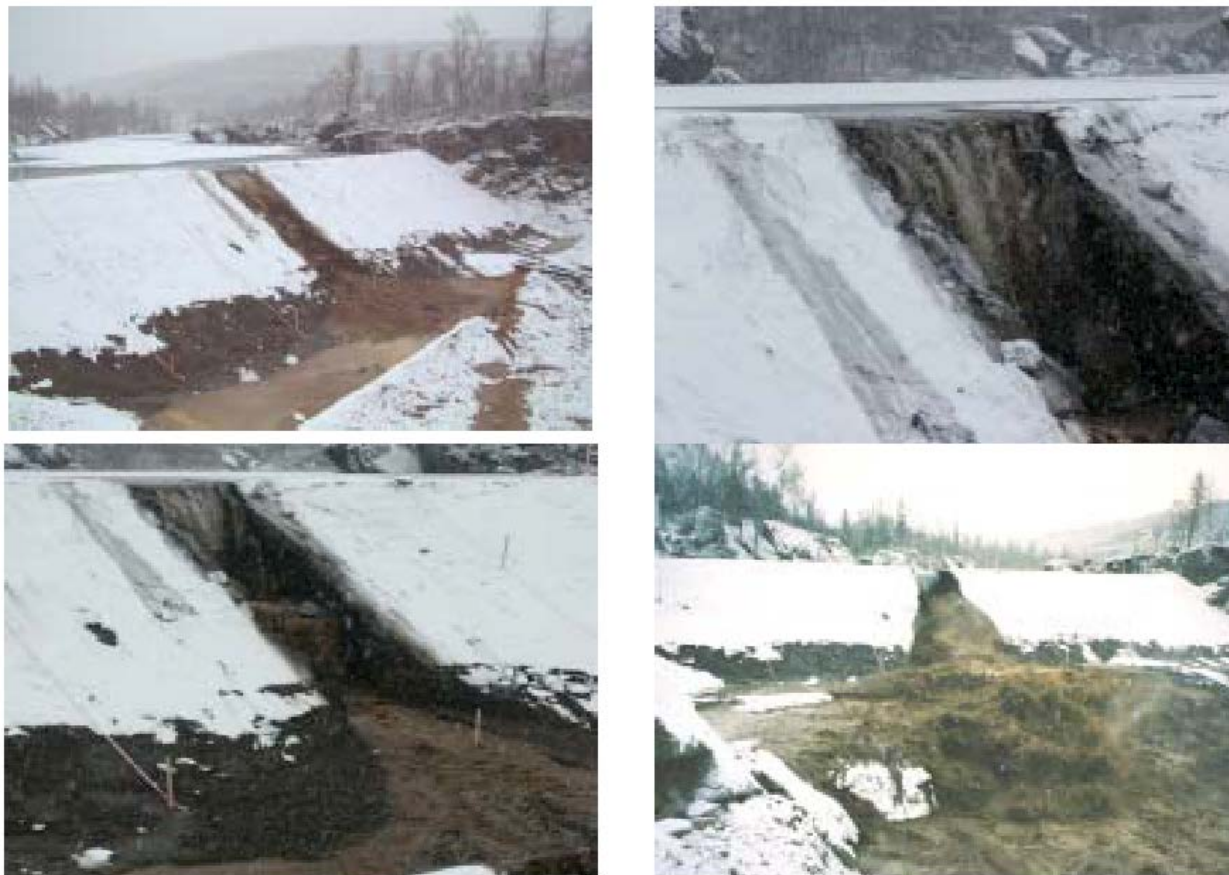
Figure 22.—Photos from the test of the Norway gravel dam, embankment 2C-02.
