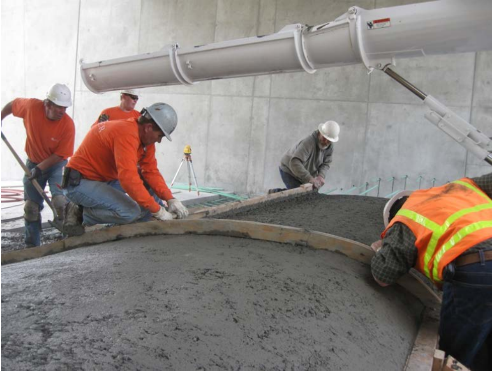
Figure 3 – Photograph showing an ogee crest placement at Scofield Dam.
