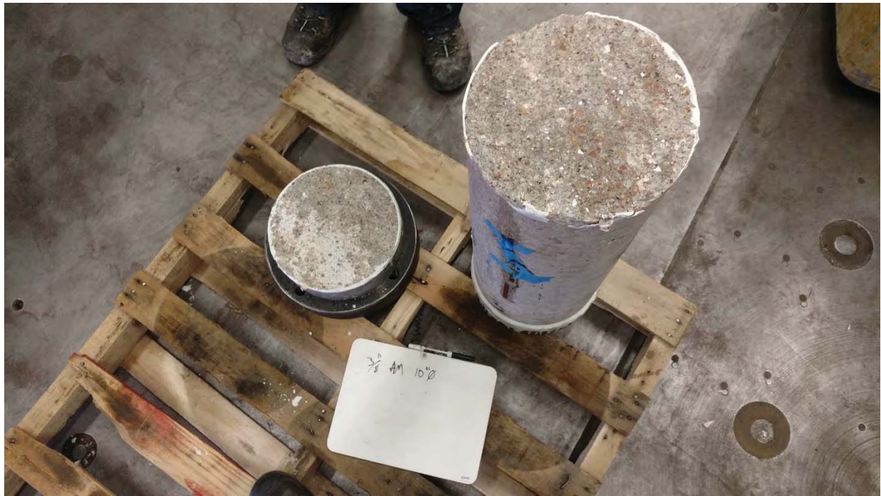
Figure I-15: 10-inch diameter core
