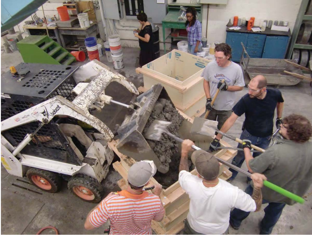
Figure D-9: Placing 8-inch NMSA concrete into forms
