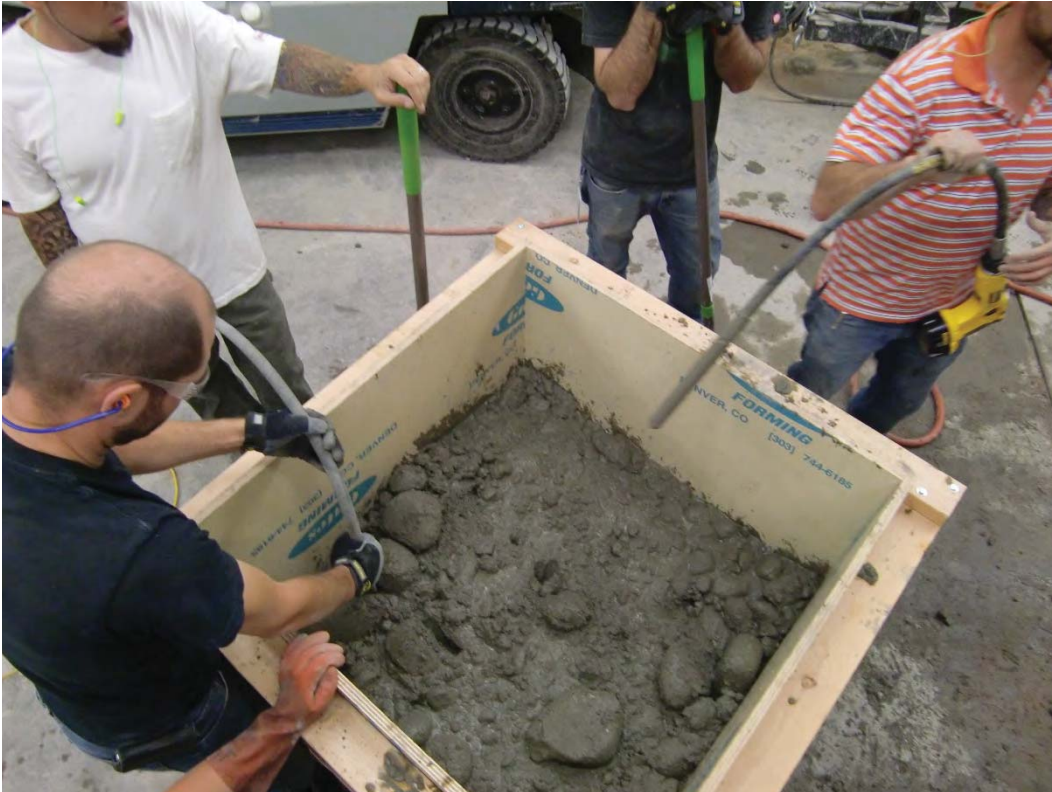
Figure D-10: Consolidating 8-inch NMSA concrete
