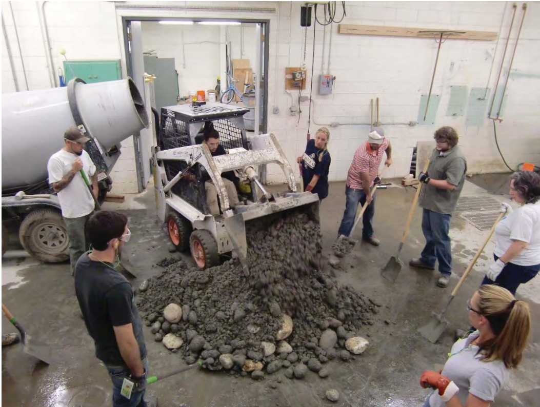
Figure D-8: Mixing 4- to 8-inch aggregate into concrete
