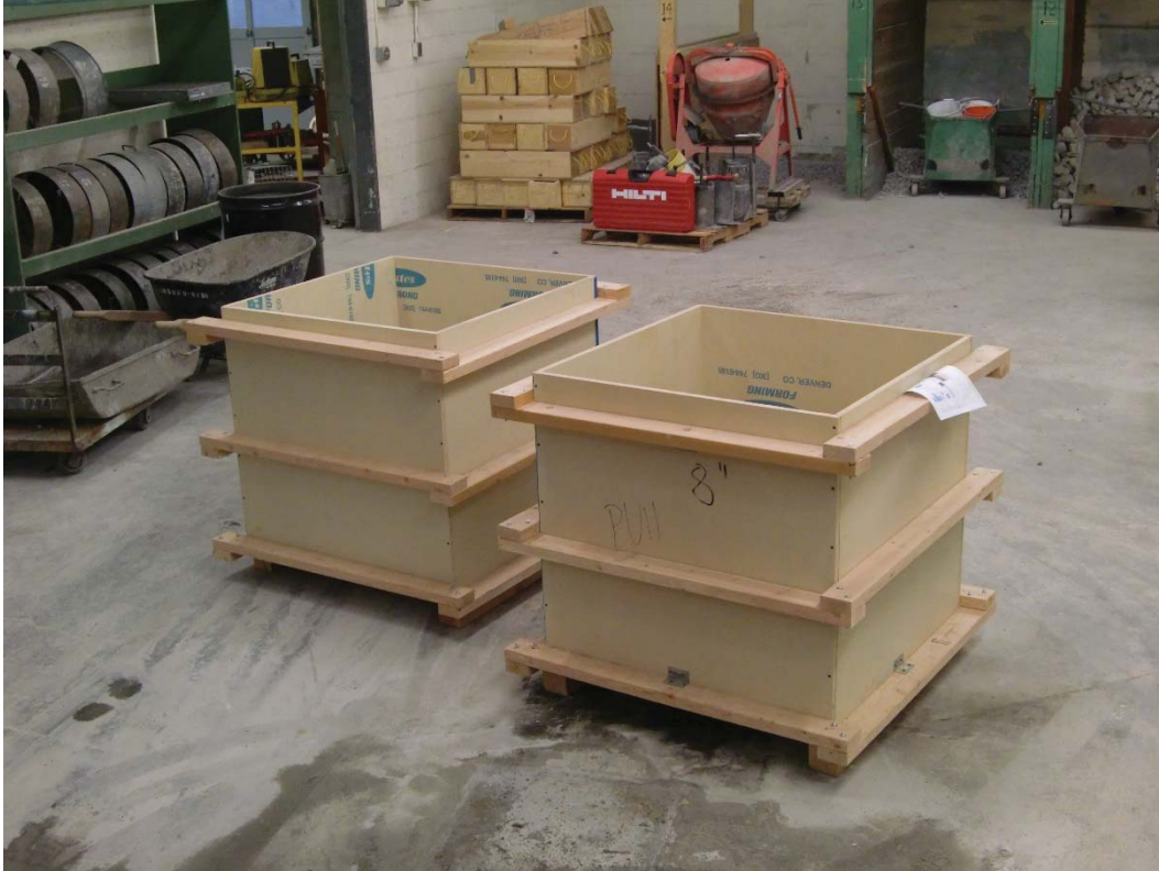
Figure 1 – Forms for 3-foot by 3-foot by 3-foot concrete blocks
