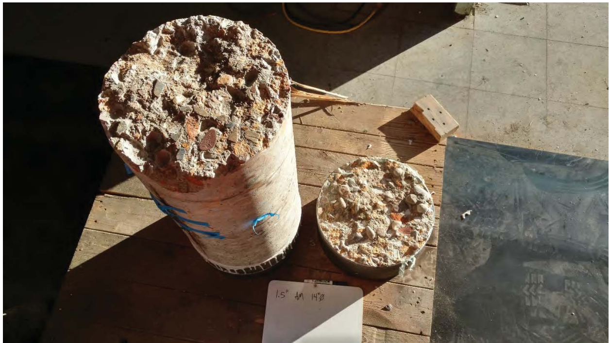
Figure I-7: 14-inch diameter core
