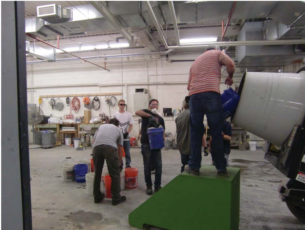
Figure D-4: Manual loading of 2- to 4-inch coarse aggregate
