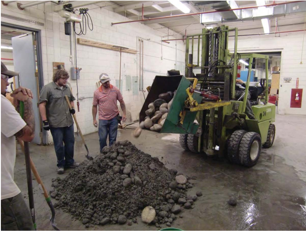
Figure D-7: Adding 4- to 8-inch coarse aggregate to concrete
