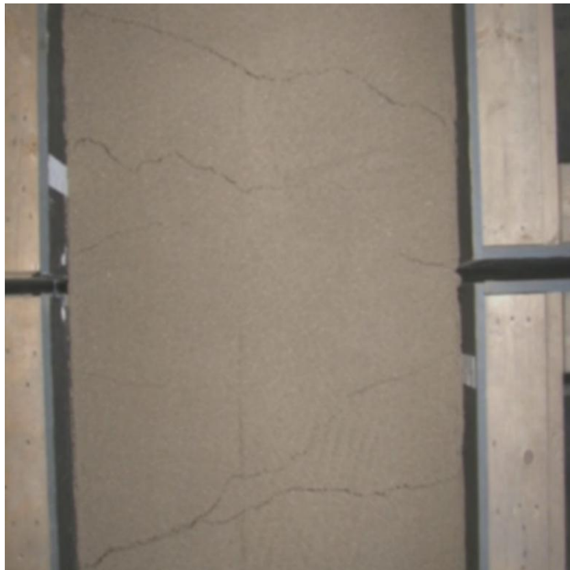
Figure 9.—Overhead view of Test 2: 3 feet of sand compacted to 81.3%.
