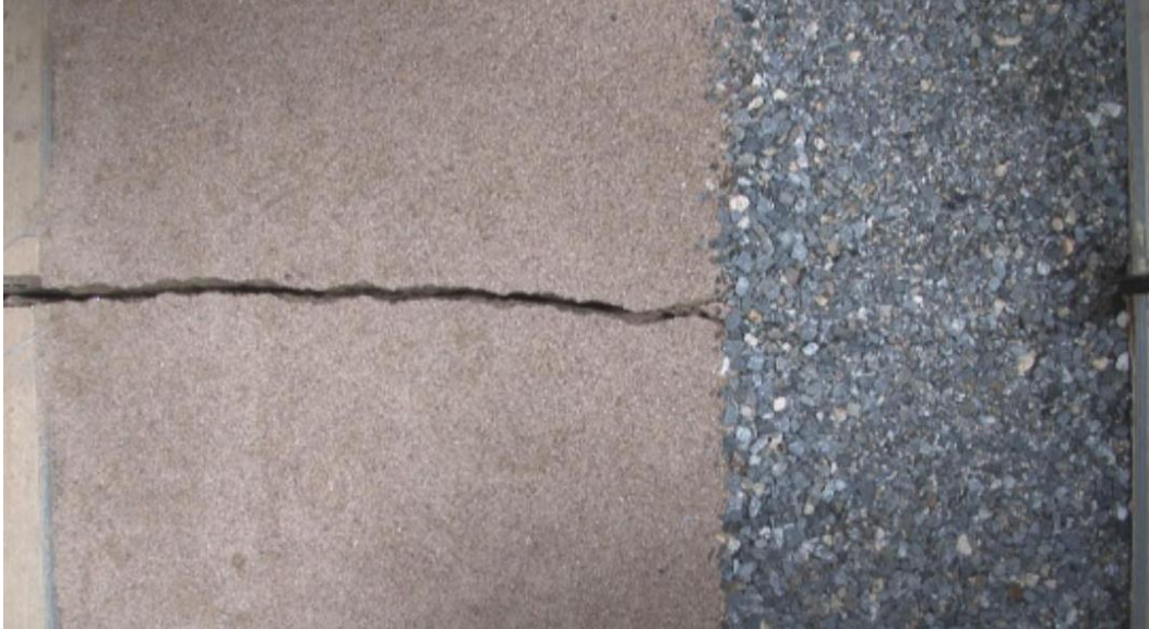
Figure 18.—Overhead view of Test 10: 3 feet of sand compacted to 91.8% and 2 feet of compacted gravel.
