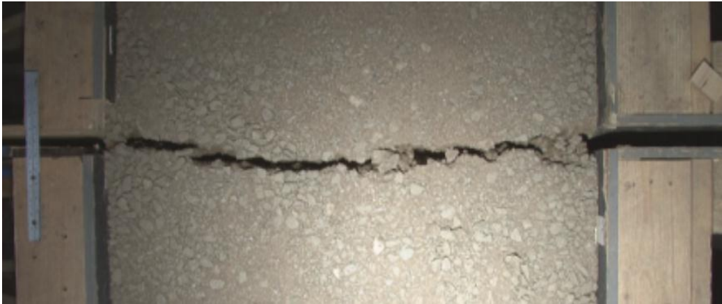
Figure 14.—Overhead view of Test 7: 3 feet of broadly graded material compacted to 94.9%.
