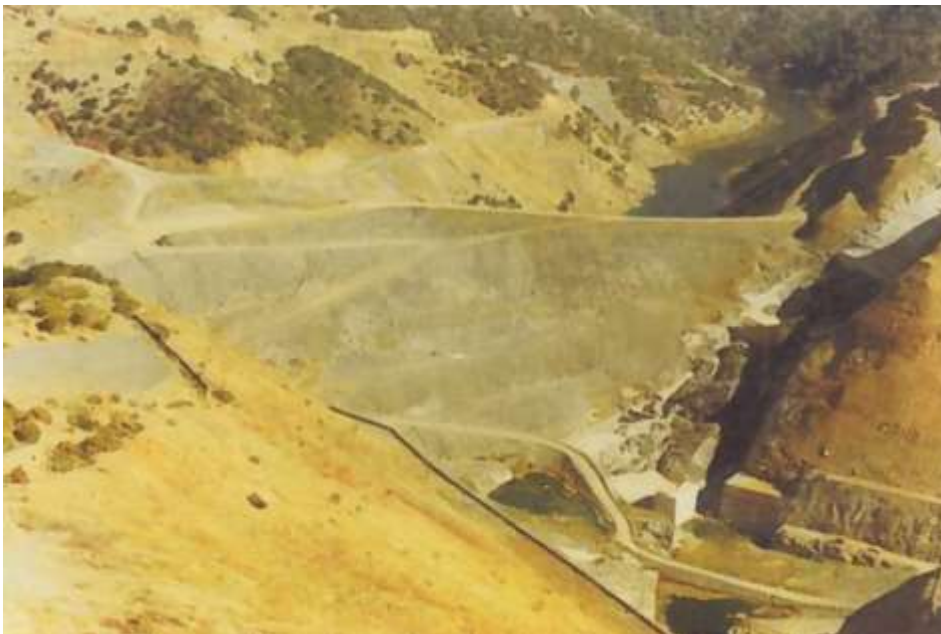
Figure A1. Aerial photo of downstream face of cofferdam.
