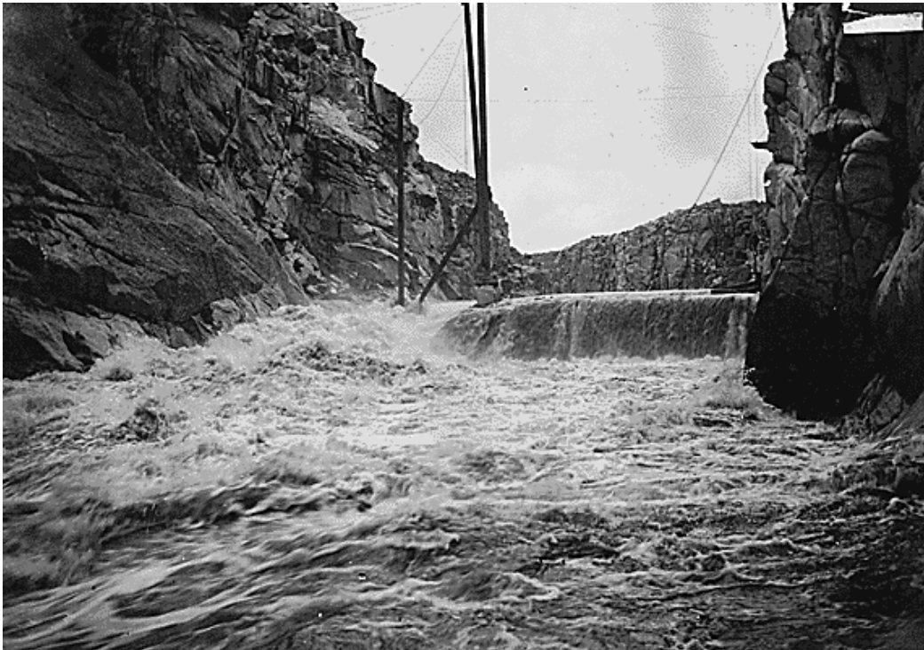
Figure 1. Partially completed masonry dam overtopping during construction.
