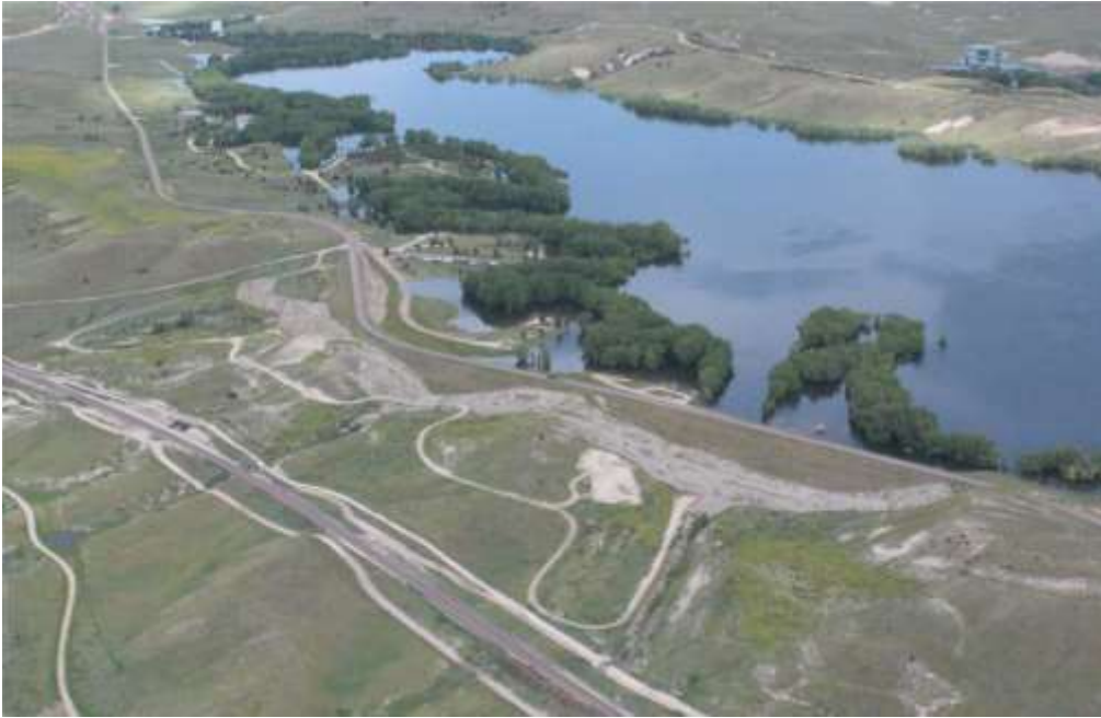
Figure 15. Aerial view of the Glendo dikes during the 2010 flood.
