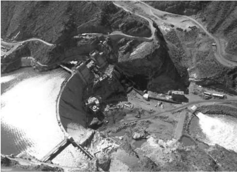
Figure 2. Photograph of Theodore Roosevelt Dam under construction, showing the cellular cofferdam, thrust block, and spillway on left abutment. This photograph shows the construction progress after the flood event.
