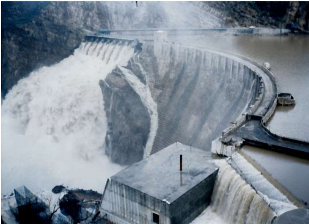
Figure 5. Theodore Roosevelt Dam during 1993 flood showing partial construction of the left thrust block and overtopping of the cellular cofferdam.
