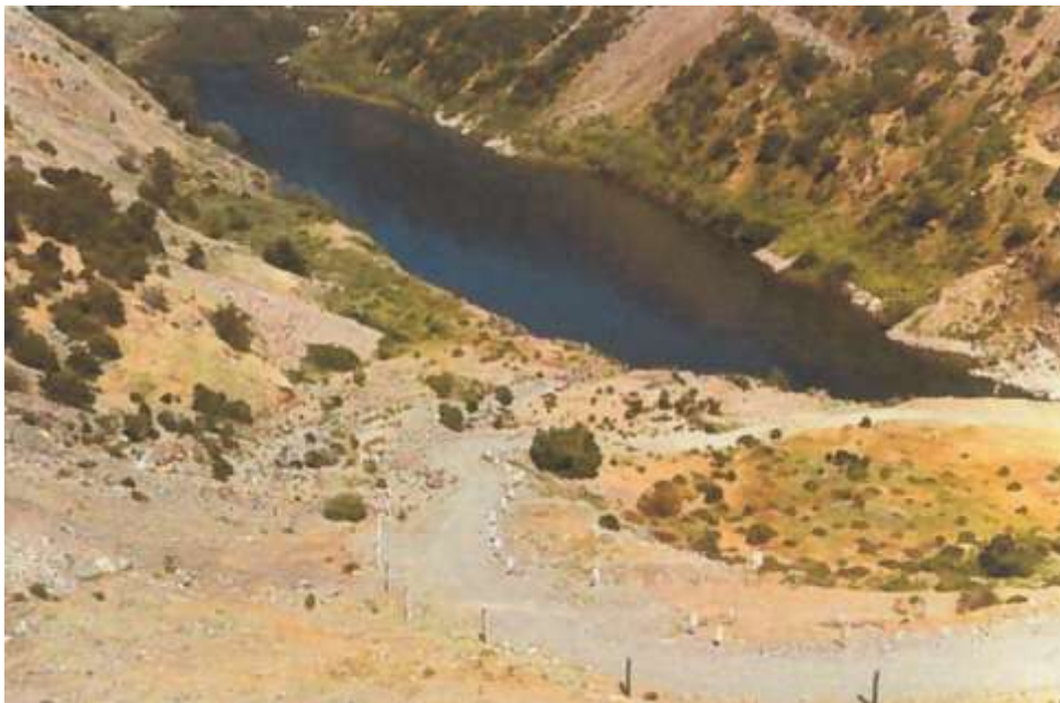
Figure A6. Photo of upstream slope of cofferdam showing markers placed every 5 feet in elevation.
