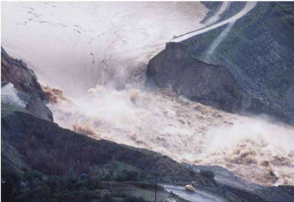
Figure A7. Aerial photograph of the cofferdam breach during the 1986 flood.
