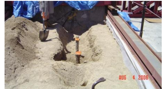
Excavating foam cores
