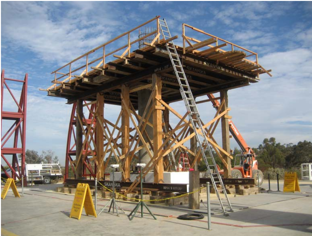
Photo 3. Construction progress of bridge on LHPOST shake table.
