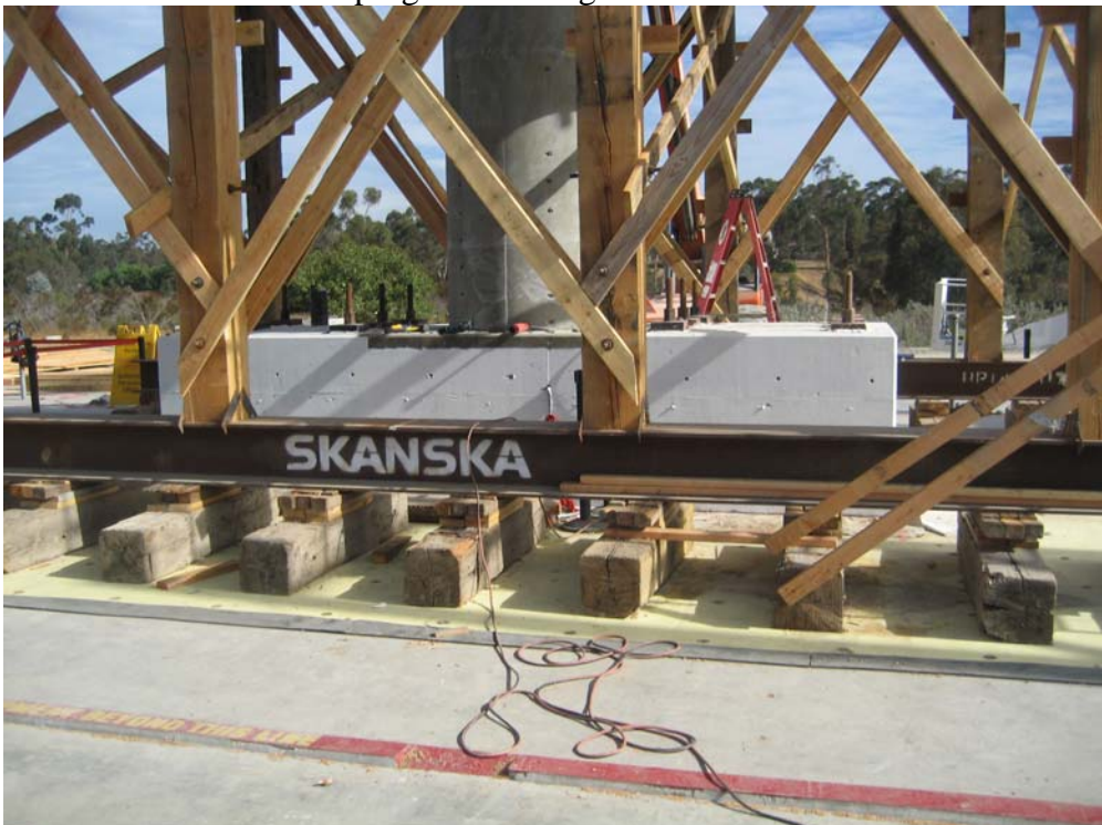
Photo 4. Close-up view of bridge pier footing connected to LHPOST shake table.
