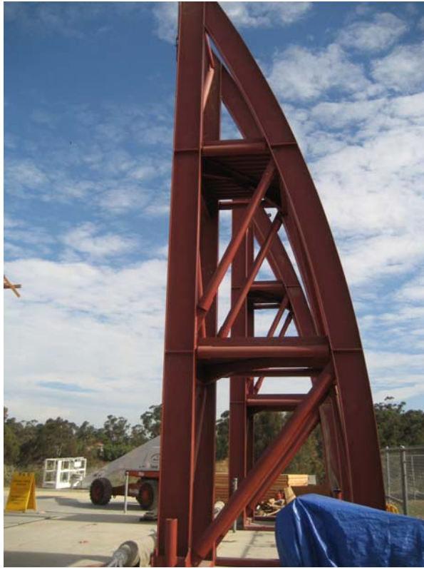
Photo 7. Steel reaction frame for future LHPOST shake table experiment.
