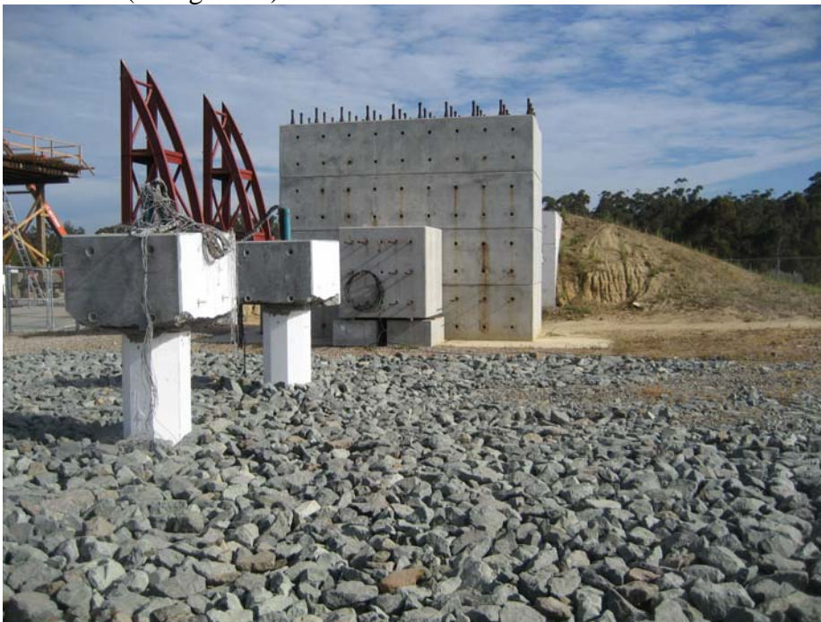
Photo 2. Close up view of soil pit with Caltran funded bridge pier surrounded by riprap.
