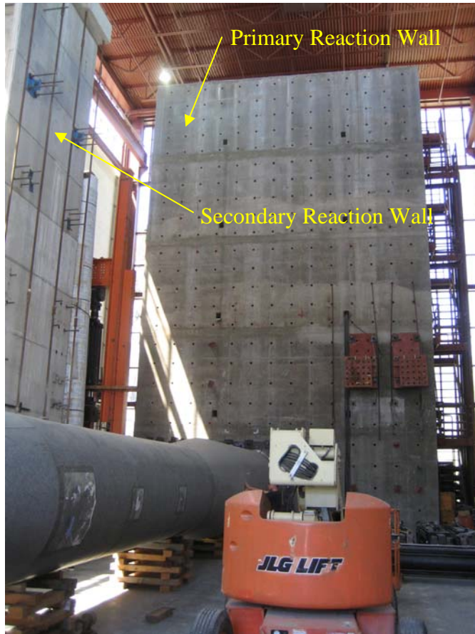
Photo 33. Reaction walls for structural testing at the UCSD La Jolla Campus facilities.
