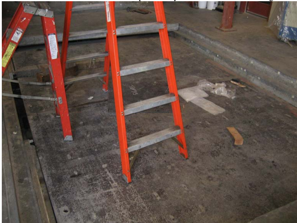
Photo 36. Small scale shake table at La Jolla Campus facility.
