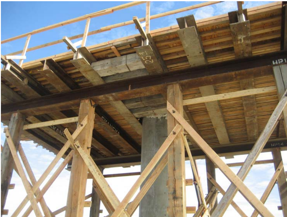
Photo 6. Scaffolding for construction of bridge pier on LHPOST shake table.
