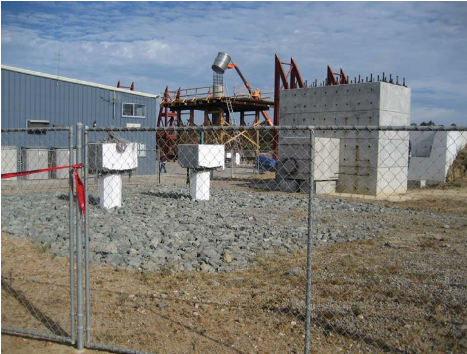
Photo 1. Soil pit experiments funded by Caltrans including testing for bridge piers surrounded by riprap (foreground) and bridge abutment foundation tests (background).
