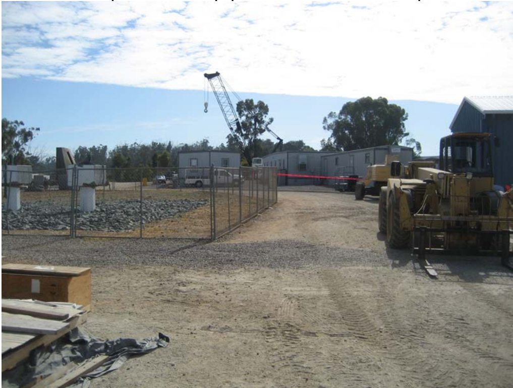
Photo 15. Office trailers for Camp Elliott.
