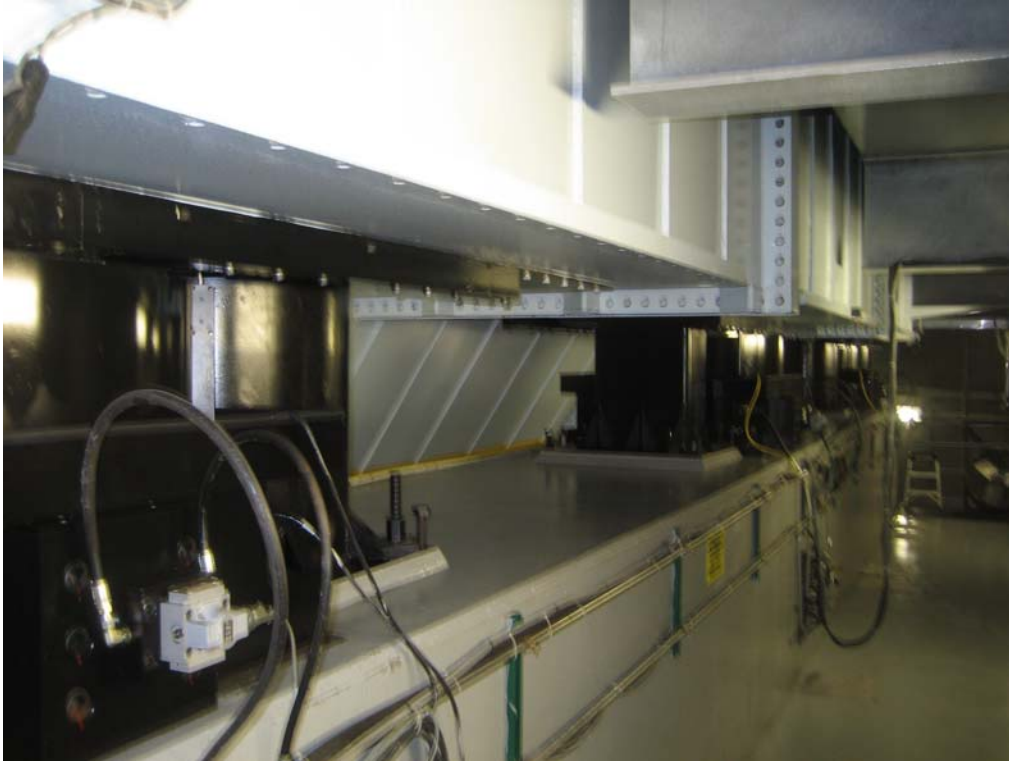
Photo 19. Hydraulic bearing supports of LHPOST shake table.
