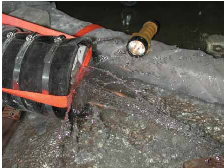
Figure 4. —Side view of a high flow of water through a cracked concrete test specimen under 3 m (10 ft) of hydraulic head before mortar injection. Flow is about 100 L/min (25 gal/min).
