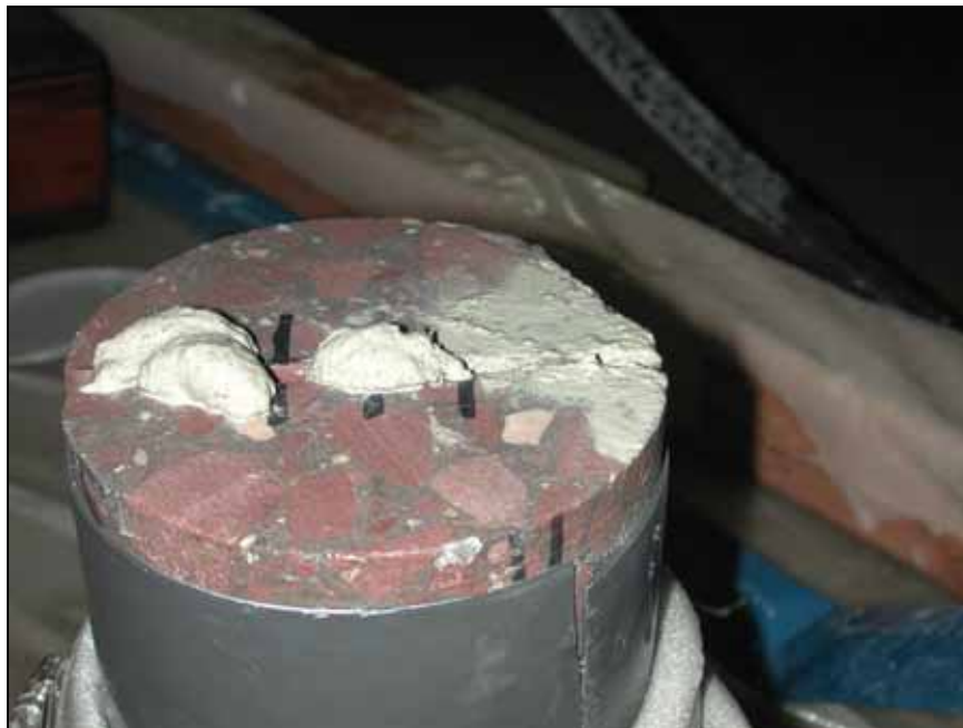
Figure 13. —First trial of underwater mortar with flow of 25 L/min filling about 25 mm (1 in) into the vertical crack face without washout. The face of the crack was filled with a second application of mortar.
