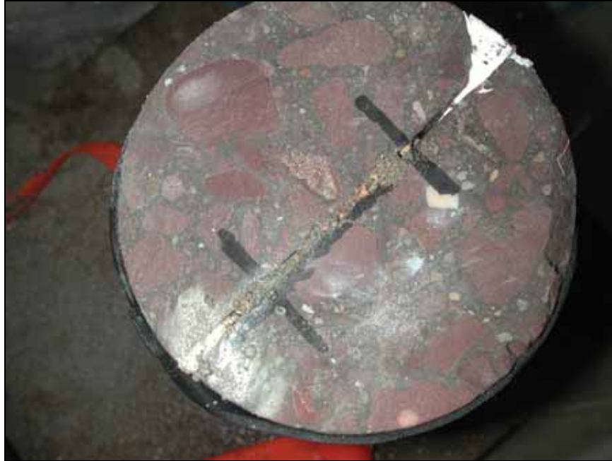
Figure 9. —3-mm ( \frac{1}{8} -in) crack filled by sand and mortar surface plugging.
