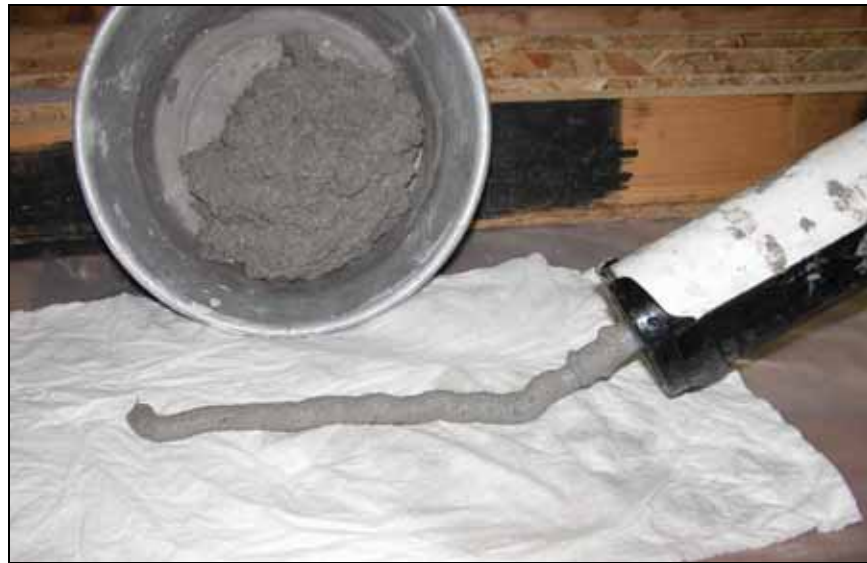
Figure 7. —Underwater crack filling mortar extruded through a caulking gun.
