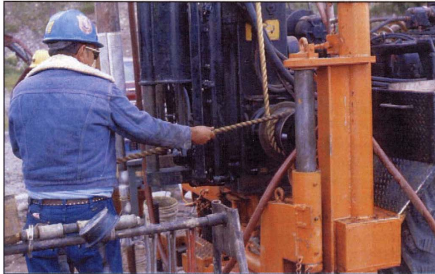
Figure 2.—Rope and cathead system for SPT.
