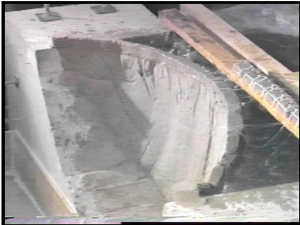
Figure 30d. —Model 11—north view, initial cracking.
