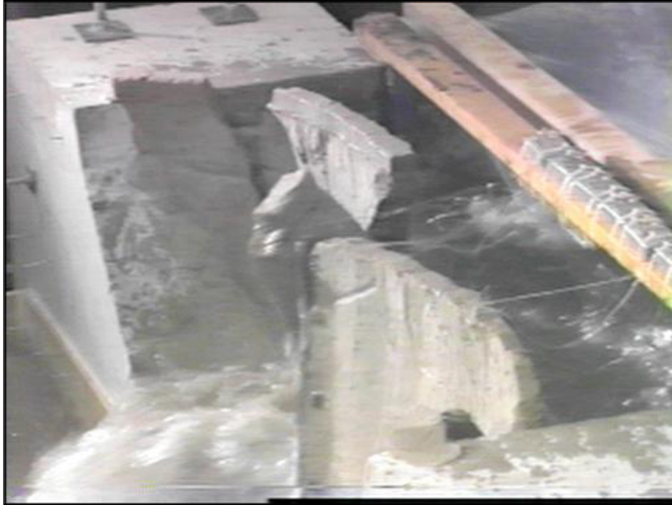
Figure 30c. —Model 11—vertical joint north view, final failure.
