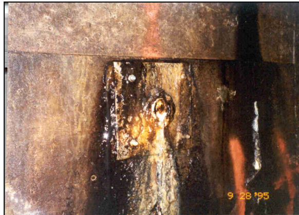
Figure 4. —The weep hole shows an example of sulfur (yellow) and phosphorous (white) related biofilm.
