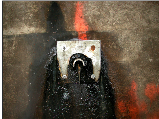
Figure 2. —The weep shows an example of a sulfate (black) related biofilm.
