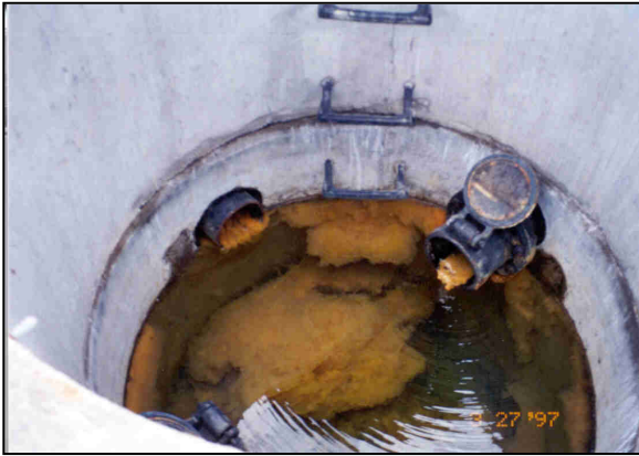
Figure 1. —The weep hole shows an example of sulfur (yellow) and phosphorous (white) related biofilm.
