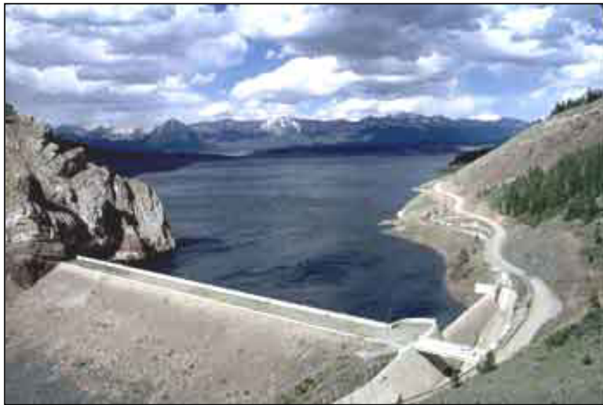
Figure 13. —Taylor Park Dam, Colorado.
