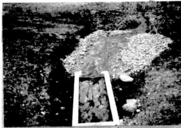
Figure 5. The weir shows an example of biofouling.
