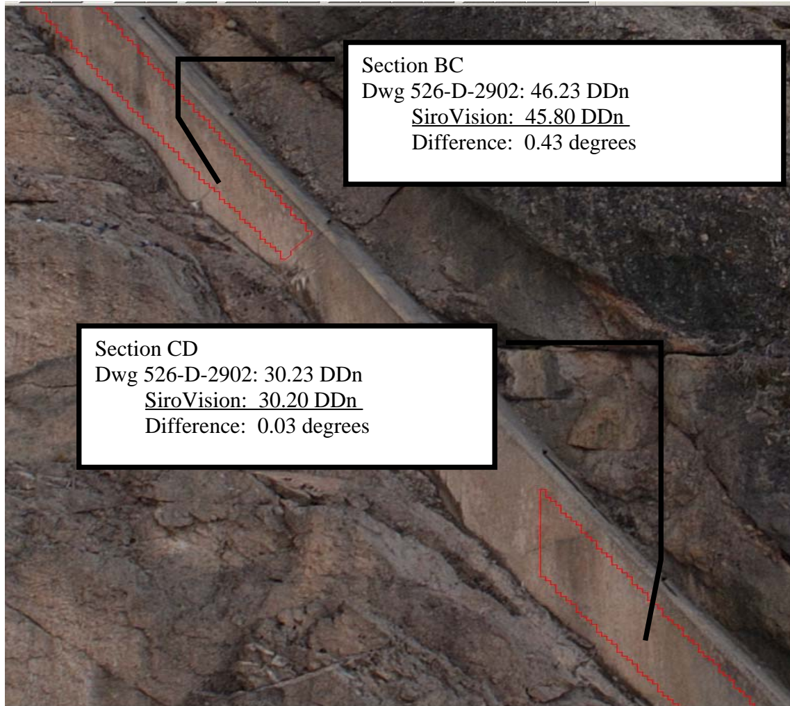
Figure A2.—Protective concrete wall, downstream left abutment, November 2002.
