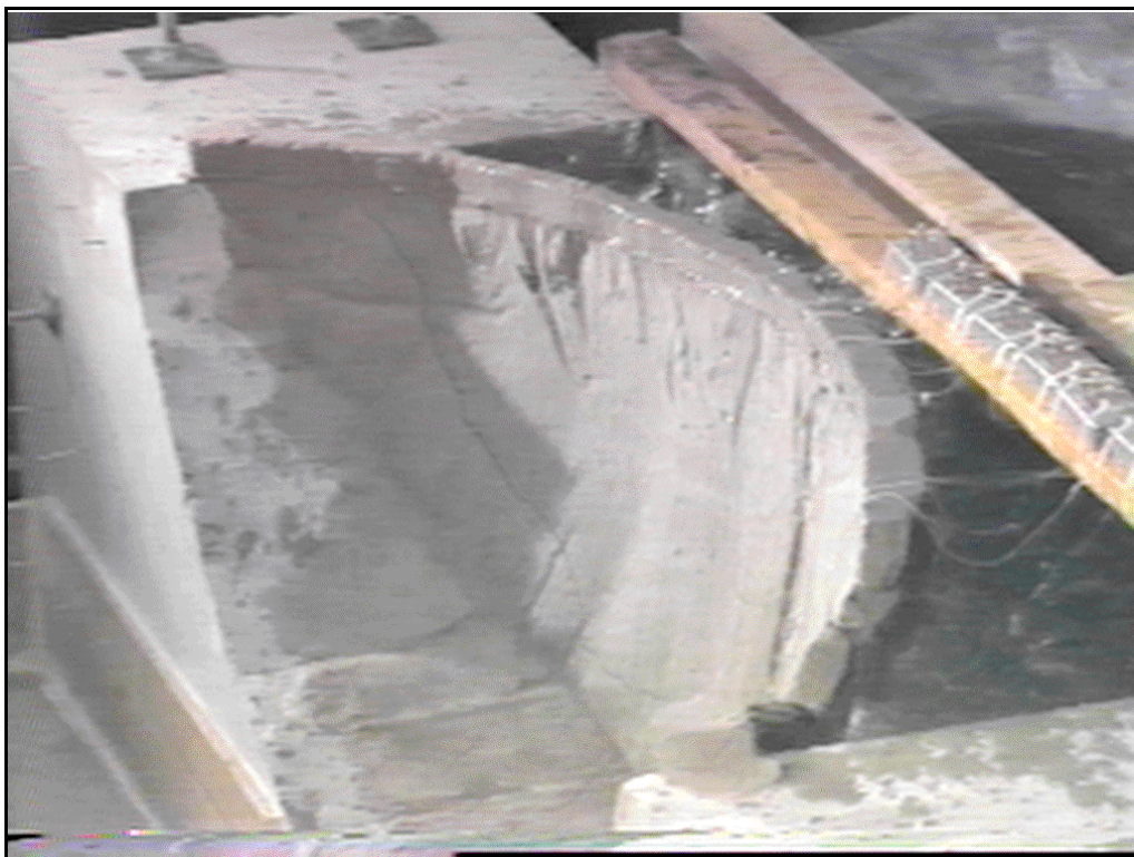
Figure 30d.—Model 11 - north view, initial cracking.
