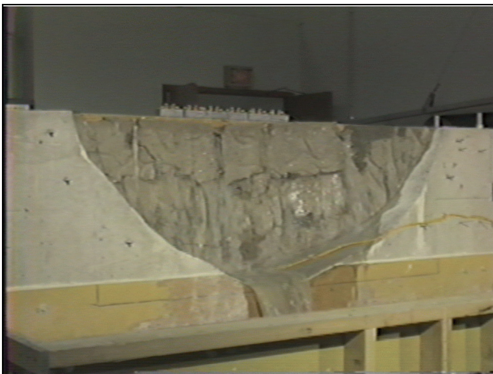
Figure 31b.—17x2 joints, final cracks.
