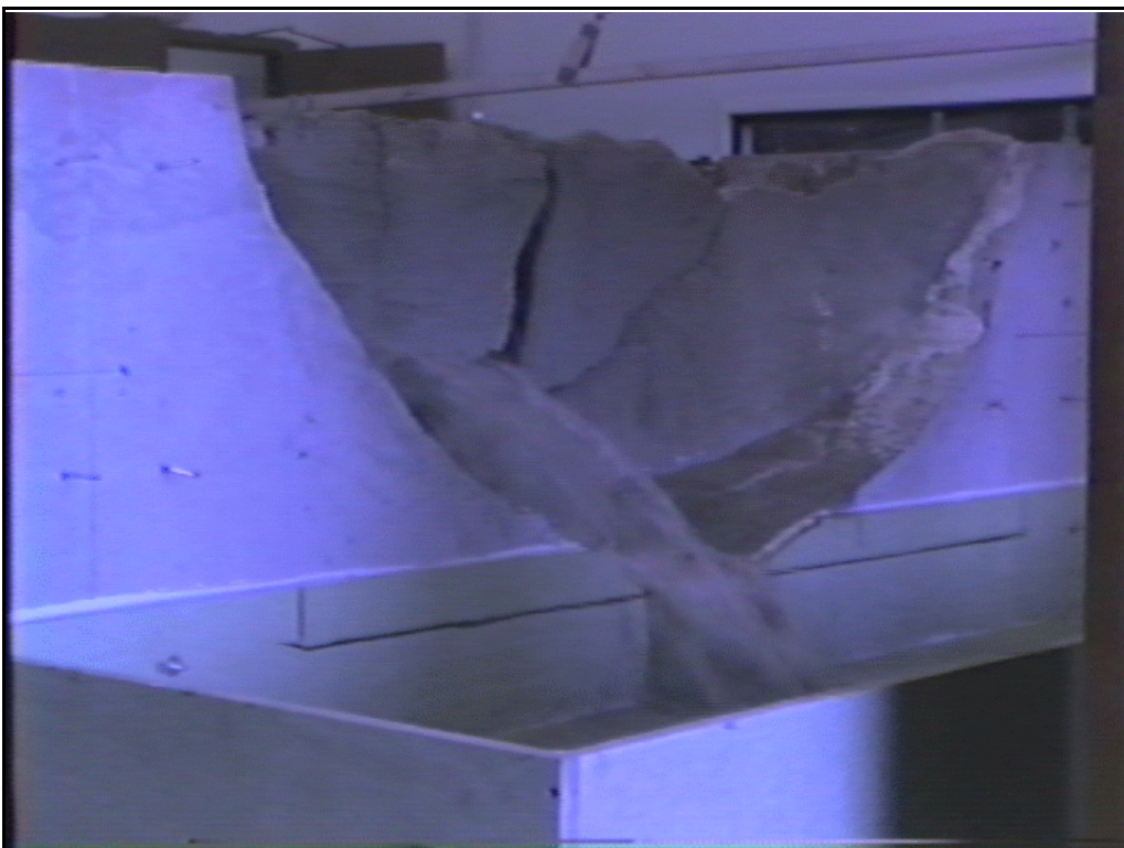
Figure 28b.— Monolithic model 2, final crack.
