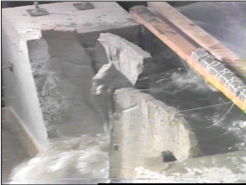
Figure 30c.—Model 11 - vertical joint north view, final failure.
