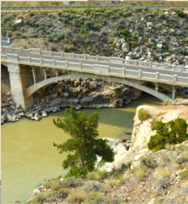
Existing Hayden Arch Bridge, Cody, Wyoming.
