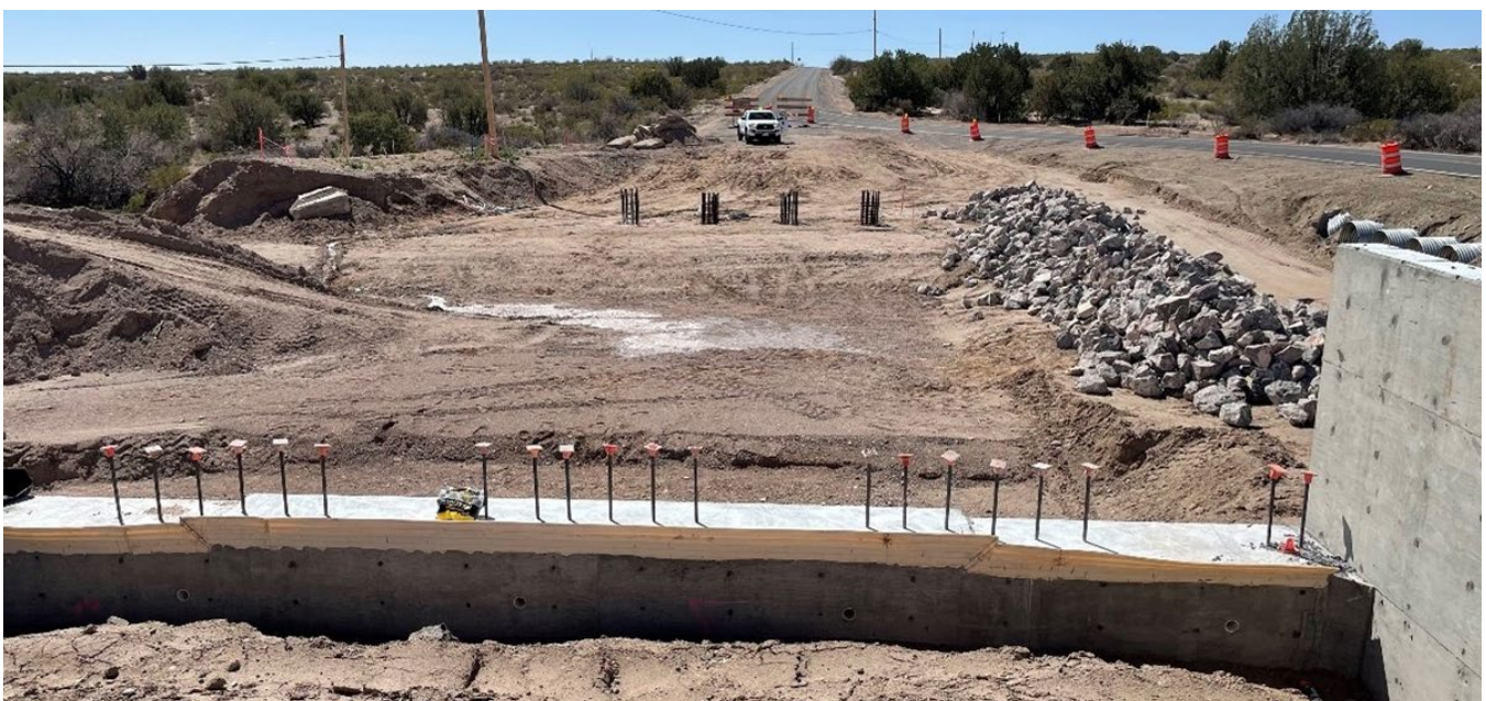
Elephant Butte Reservoir Lakeshore Road Site 4 bridge construction, New Mexico.
