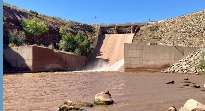
Sumner Spillway Bridge, New Mexico.
