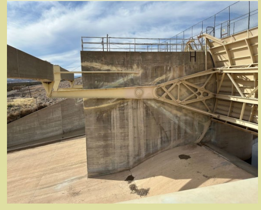
Caballo Dam, New Mexico, spillway radial gate.
