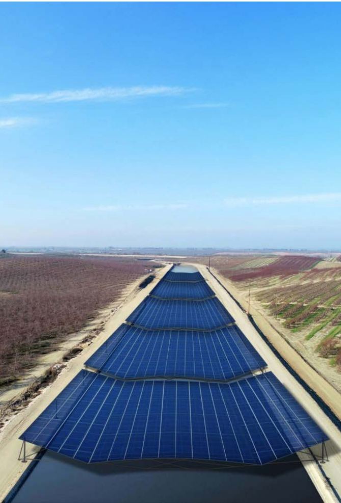
Conceptual rendering of solar panels spanning the 110 foot-wide Turlock Irrigation District Main Canal, California (Solar AquaGrid LLC).
