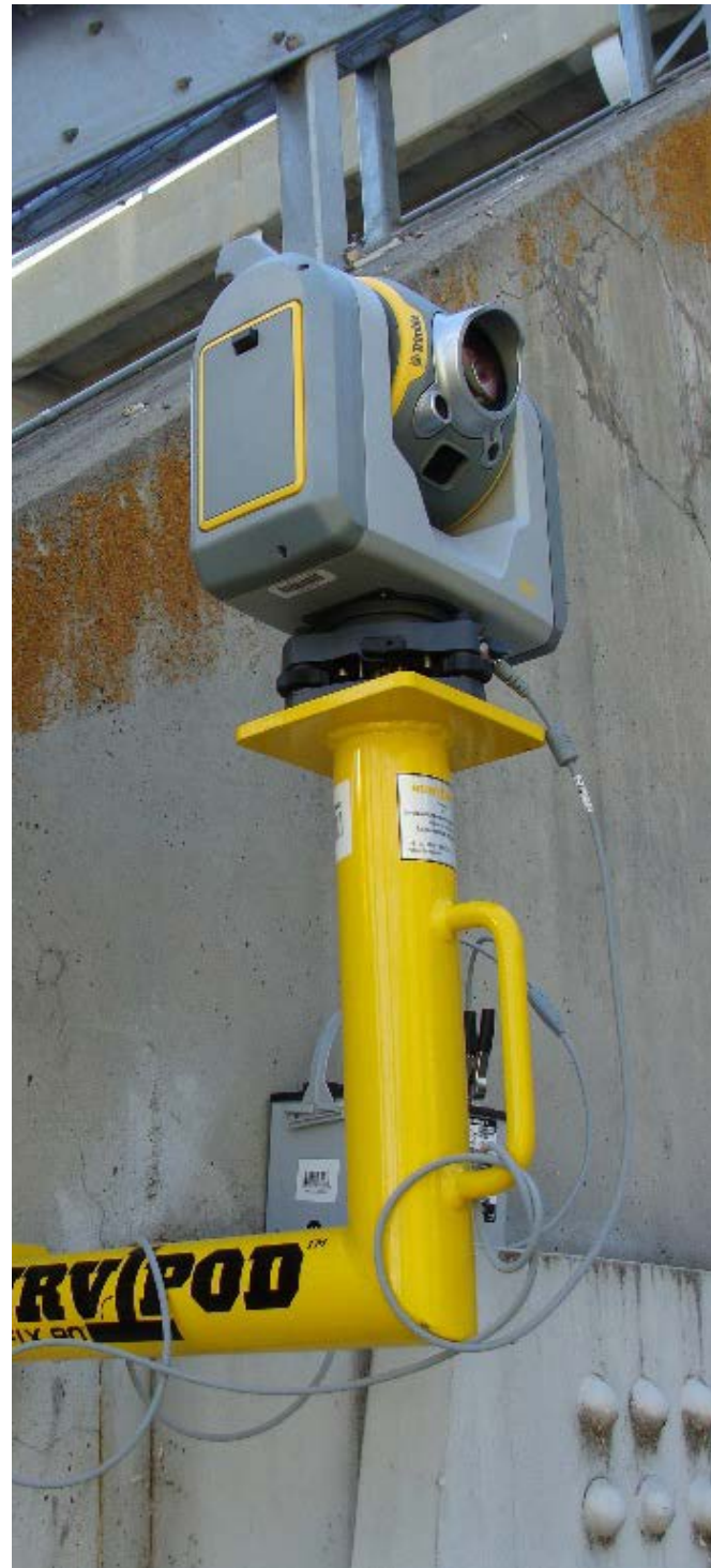
Scanning and imaging the radial gates at Canyon Ferry Dam, Montana.
