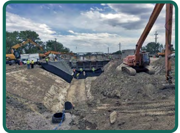
Reclamation and TCID installing geotextile liner during the repair operations.
