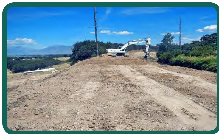
Finished canal embankment— 8/28/2015.
