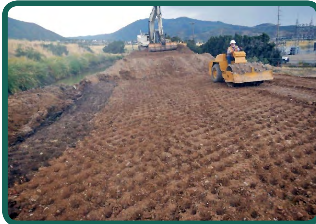
Backfill operations showing neat line of clay liner and fill material—8/27/2015.
