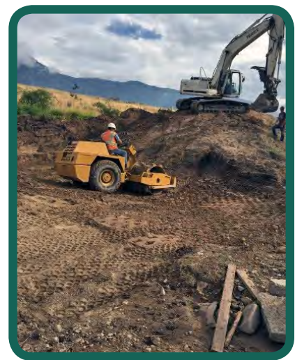
Compacting the embankment foundation after excavating the emergency repair fill material.
