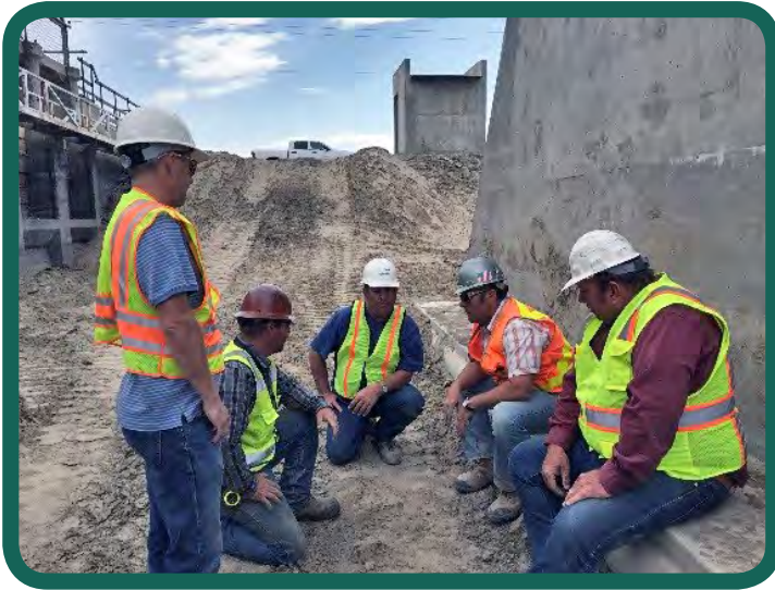
Reclamation and TCID discussing the next phase of the repairs.
