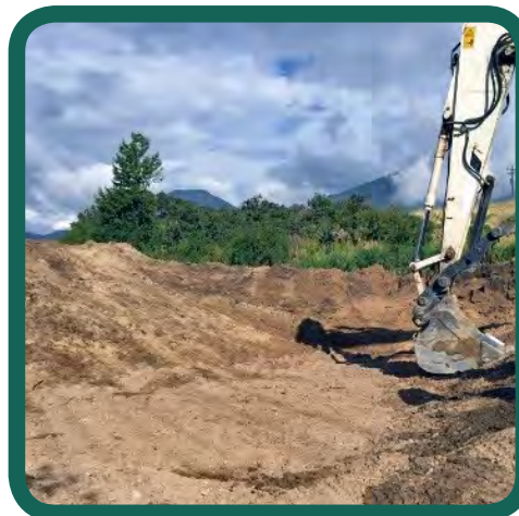
Compacting the embankment foundation after excavating the emergency repair fill material.
