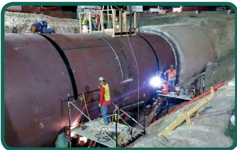
Welders working outside the siphon piping right of centerline.
